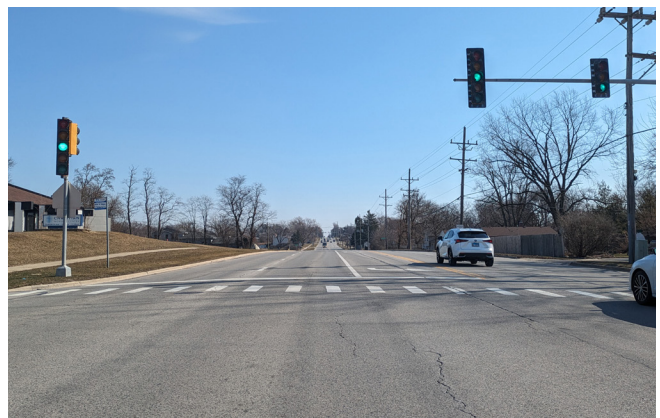
63rd Street at Dunham Road Source: Baxter & Woodman
