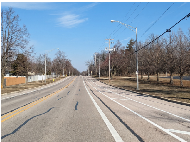
Dunham Road bicycle lane at O'Brien Park Source: Baxter & Woodman
