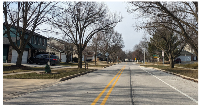
Concord Drive at Bunker Hill Circle Source: Baxter & Woodman
