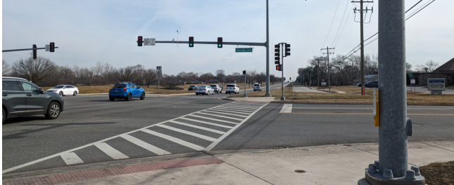
Southern DuPage County Regional Trail, Fairview Avenue
