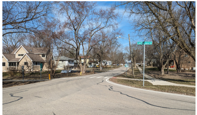
Southern DuPage County Regional Trail Crossing
