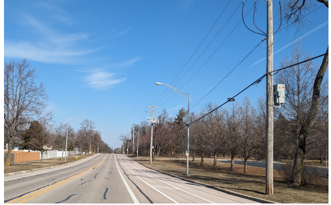
Dunham Road buffered on-street bicycle lane at O'Brien Park
