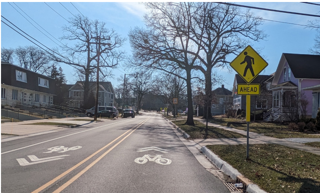
Sharrows on Carpenter Street
