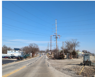
Rail crossing conditions at Maple Avenue
