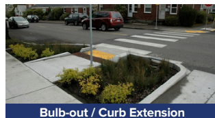
Bulb-out / Curb Extension
