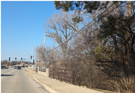
Bridge along Belmont Avenue
