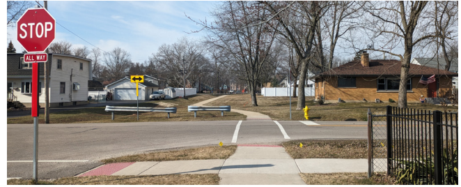
New ADA compliant crossings
