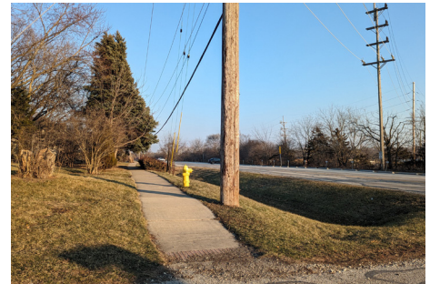
Debris and buckling on Warren Avenue
